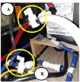
Water Heater Bypass Valves (shown in bypass mode)
